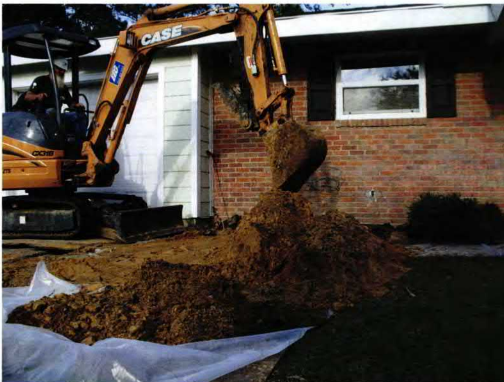
Picture 2: UST 511LaurelBB excavation in progress.
